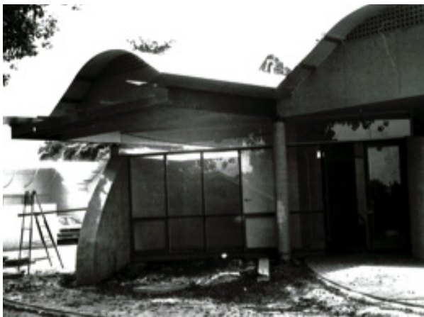
Sophia under construction in 1990
